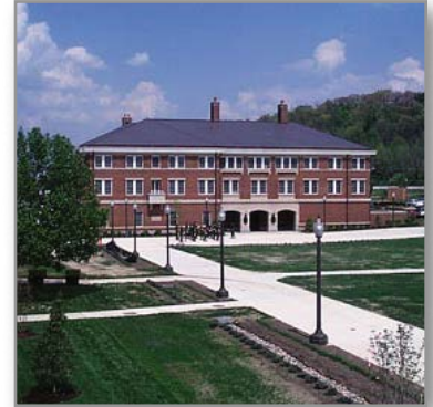
Federal uses occupy a range of physical settings, from self-contained enclaves like Bolling Air Force Base to grand office buildings in the heart of Downtown Washington.
