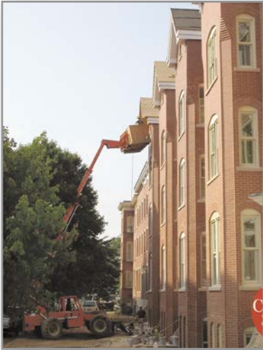
7th Street NE rowhouses under construction
